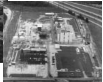
CertainTeed's ISO 9000-certified PVC resin manufacturing plant in Sulphur, Louisiana.
