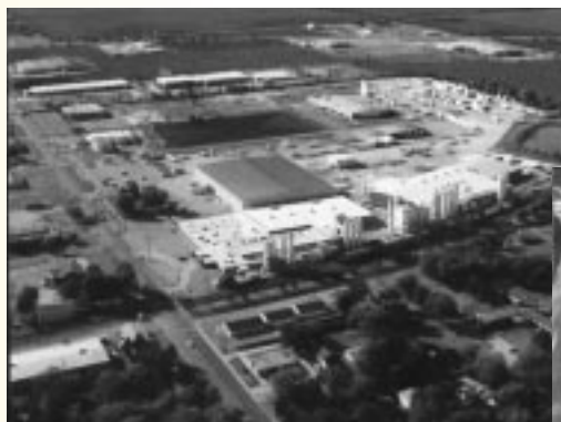
Our extrusion and molded plastic production plants in McPherson, Kansas, where Yelomine™ pipe and couplings are manufactured.
